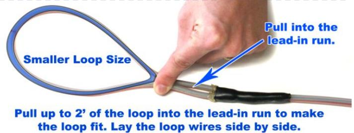
**Pull up to 2' of the loop into the lead-in run to make the loop fit. Lay the loop wires side by side.**
